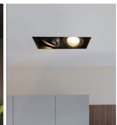
New black double lights to ceiling
