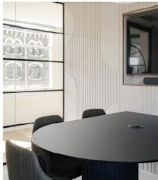
Acoustic panels to meeting rooms
