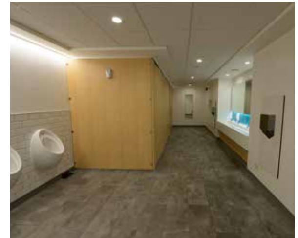
Newly refurbished WC's
