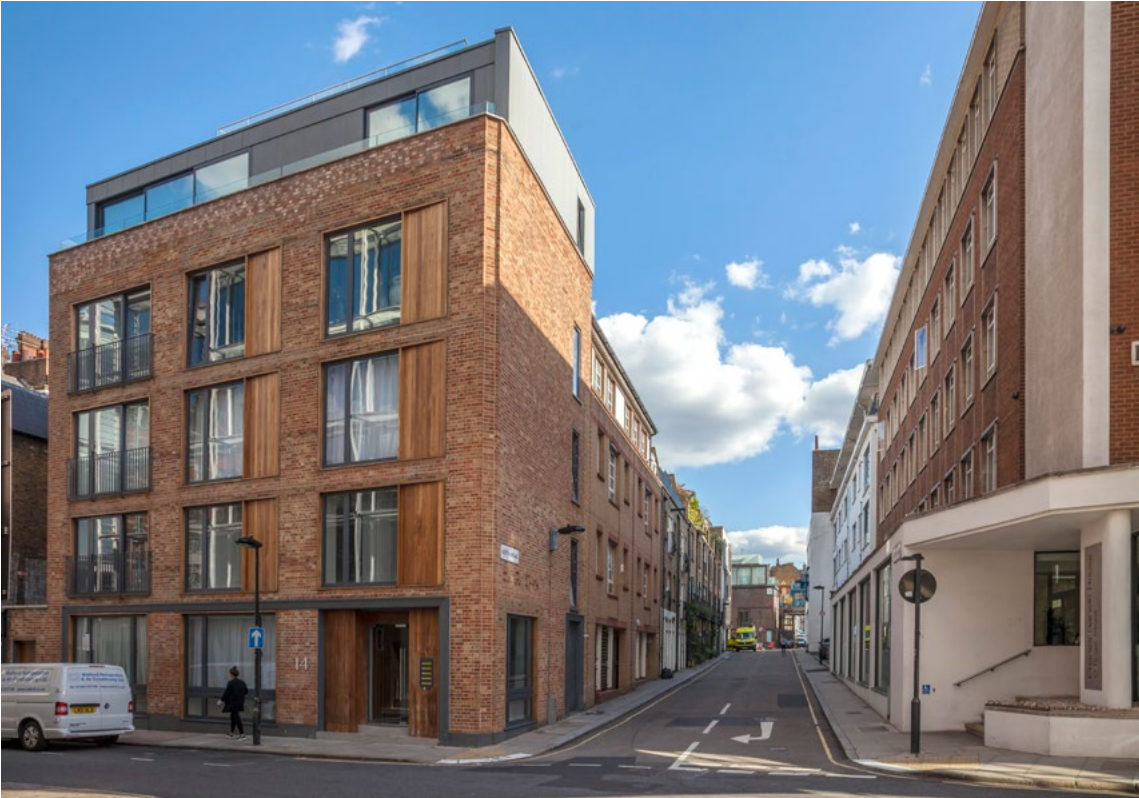
Additional floor at 14 Roger Street opposite Charles Darwin House
