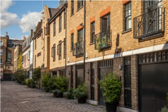
Local residential properties in Brownlow Mews adjacent to Charles Darwin House
