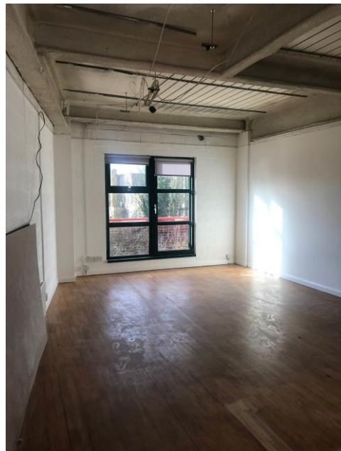
Stripped out and being re fitted
