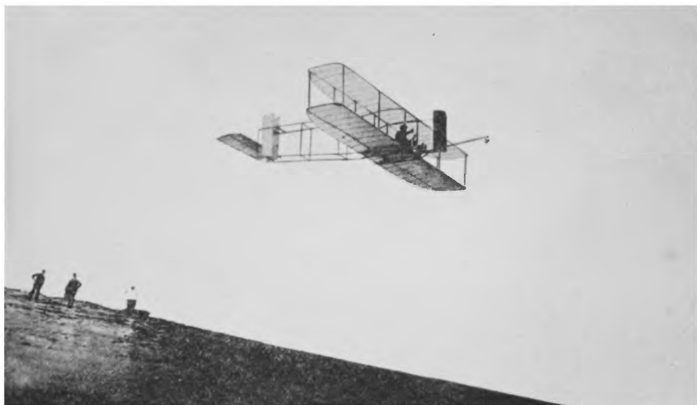
FIG. 16.—The Wright glider of 1911. This glider, in which a record was set, has a control system very similar to the one used at present.
