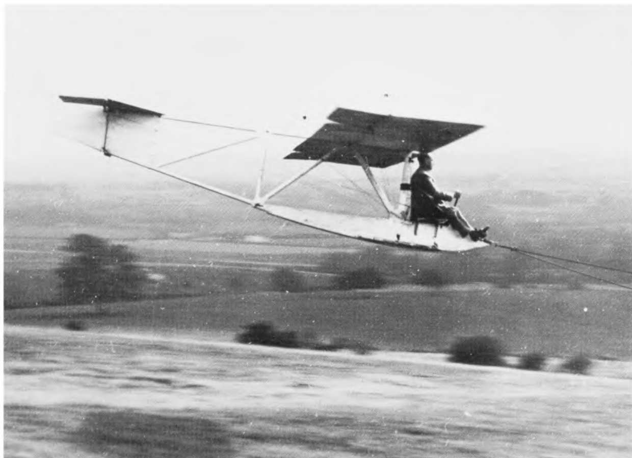
Zogling glider being catapult launched at Dunstable. (Aeroplane Monthly).
