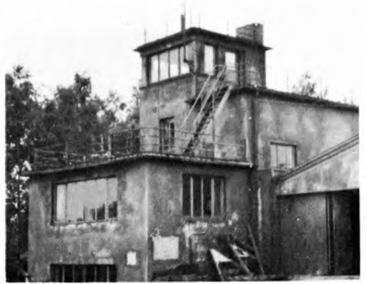
Control Tower at Oerlinghausen.
