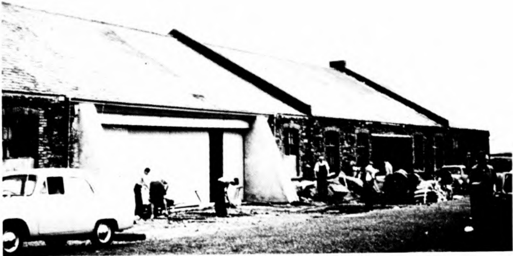
Members building the entrance to the first hangar.
