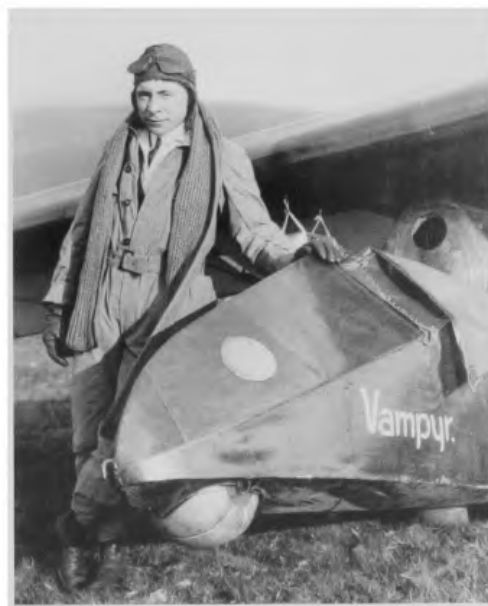
The Vampyr, showing the pneumatic, tricycle undercarriage and the leather cockpit cover which was fastened over the pilot's shoulders, leaving only his head exposed. The pilot here is Hentzen.
