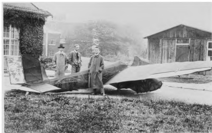
Above: The FVA - 1 Schwatze Düvel under construction in the workshop of the Aachen Technical University. The deep wing profile at the root allowed the strong but very light spars to be fully enclosed without external struts or bracing wires.
