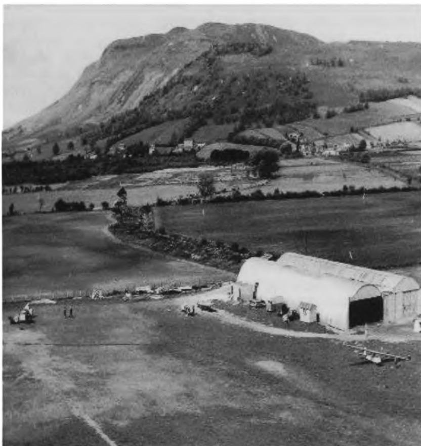
The Hangar with toilet block at the far end and the Bishop Hill Hut bits near the far fence, awaiting assembly. Bishop Hill is in the background.
