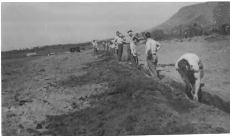
Digging the foundations for the hangar
