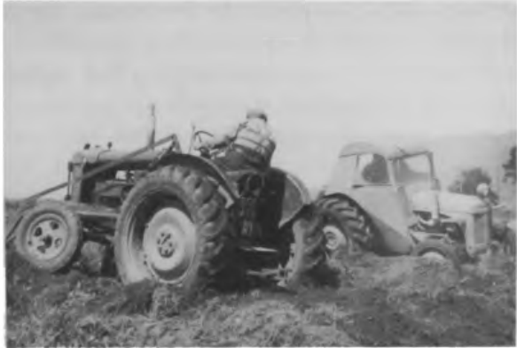
Levelling the site for the hangar.
