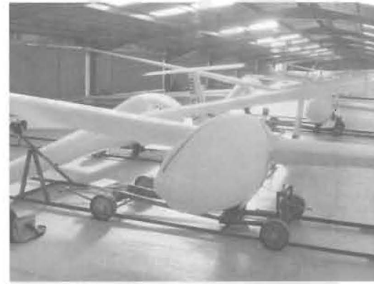
The new 22-glider hangar at Borders GC, Milfield
