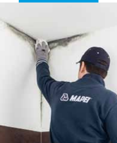
Cleaning the walls with Silanolor Cleaner Plus
