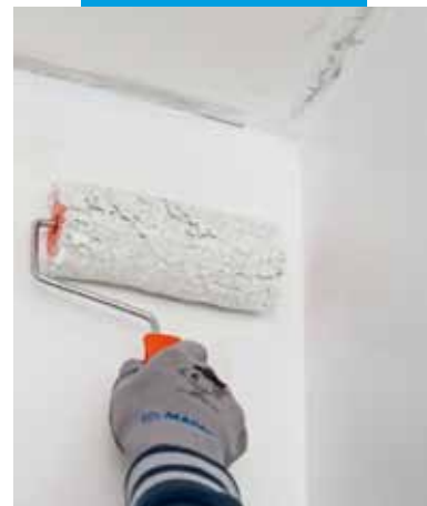
Application of Dursilite Plus with a roller
