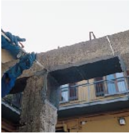
Repairing beam with injection of EPOJET
