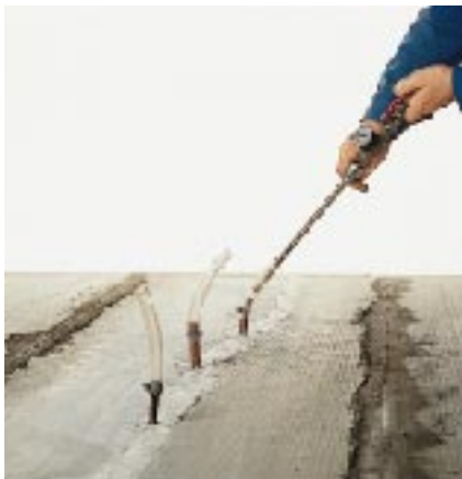
Restoring horizontal structure by injection with EPOJET
