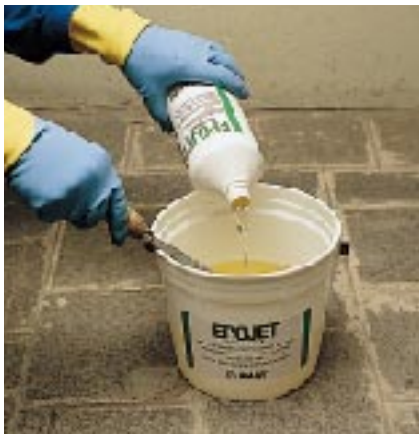
Mixing the 2 components of EPOJET
