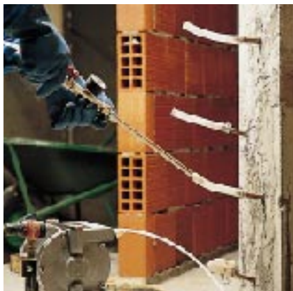
Injecting EPOJET to a fissured pillar
