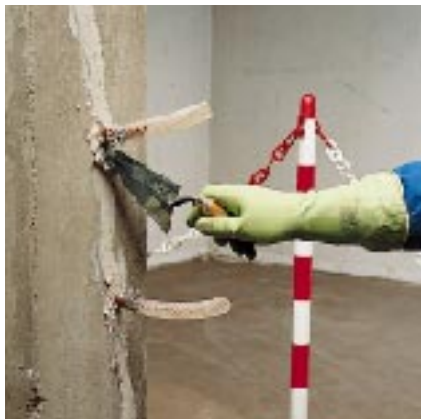
Fixing injection tubes with ADESILEX PG1
