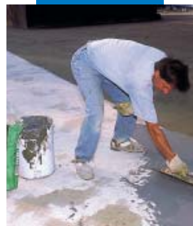
Waterproofing of a swimming pool with Mapelastic
