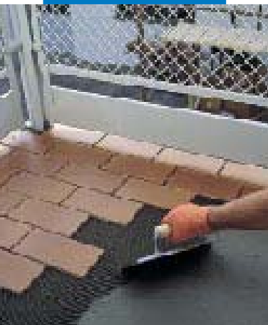
Setting tiles with Granirapid onto a balcony waterproofed with Mapelastic
