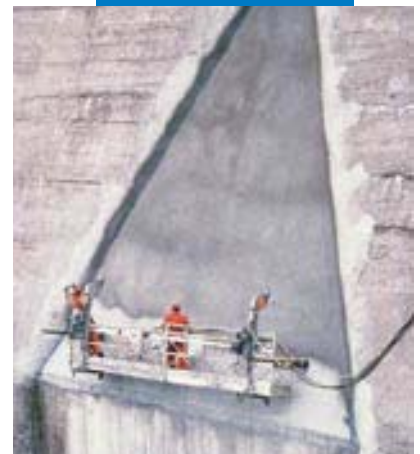
Example of Mapelast applied on a dam by spraying
