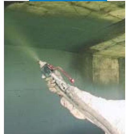
Example of Mapelast applied on a viaduct by spraying
