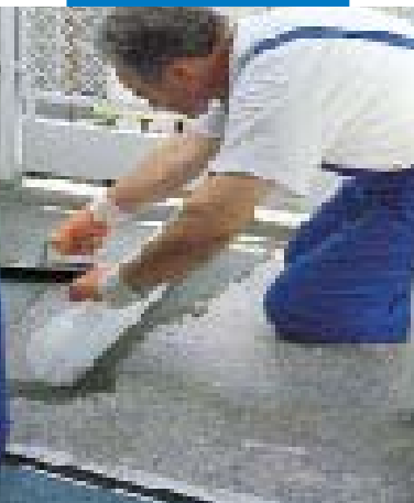
Waterproofing a balcony with Mapelastic incorporating a fibreglass net reinforcement
