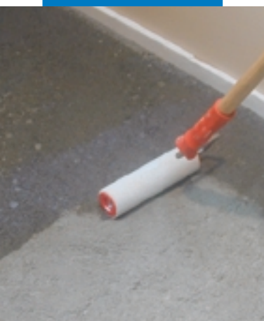
Applying Primer G with a roller
