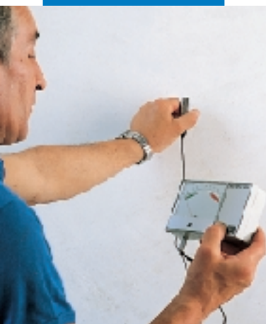
Checking plaster humidity
