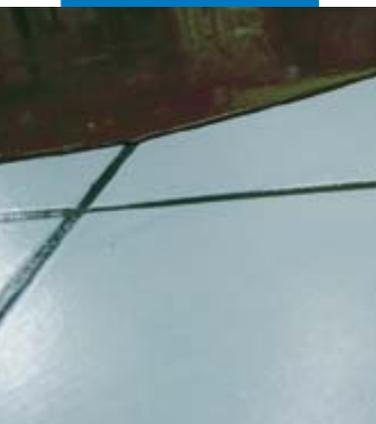
Detail of the application of Ultraplan on an existing ceramic tile floor after the application of Mapeprim SP
