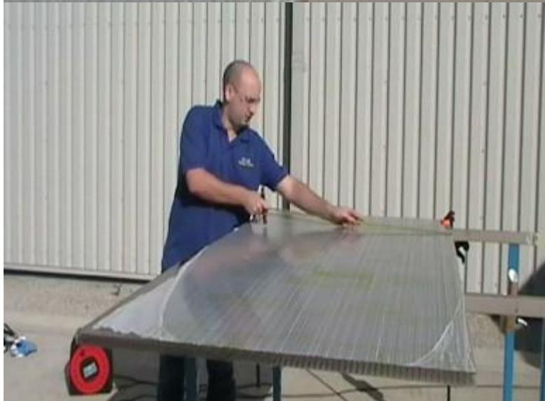
4. Mark the centre of the sheet, ready to cut the hole for the vent.
