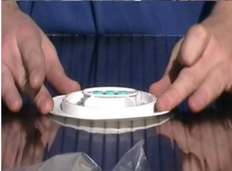
18. The vent is now installed into the sheet ready for the sheet to be installed into the roof.
