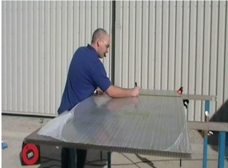
5. A 114mm hole saw is required for cutting the hole into the polycarbonate roof sheet.
