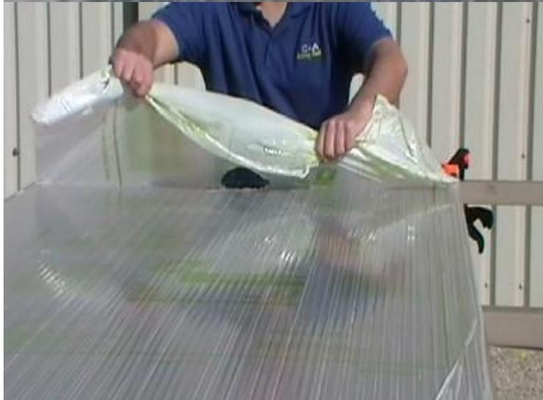
9. When securing the sheet, we recommend that only Stixall adhesive is used to ensure a good adhesion and water tight seal.
