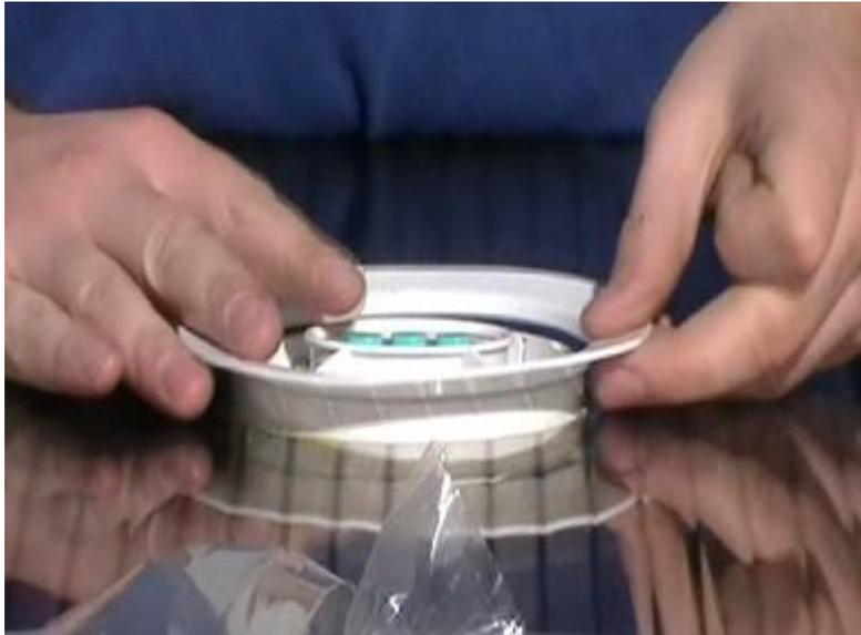
17. Push the vanity plate until it is firmly on the underside of the polycarbonate roof sheet.
