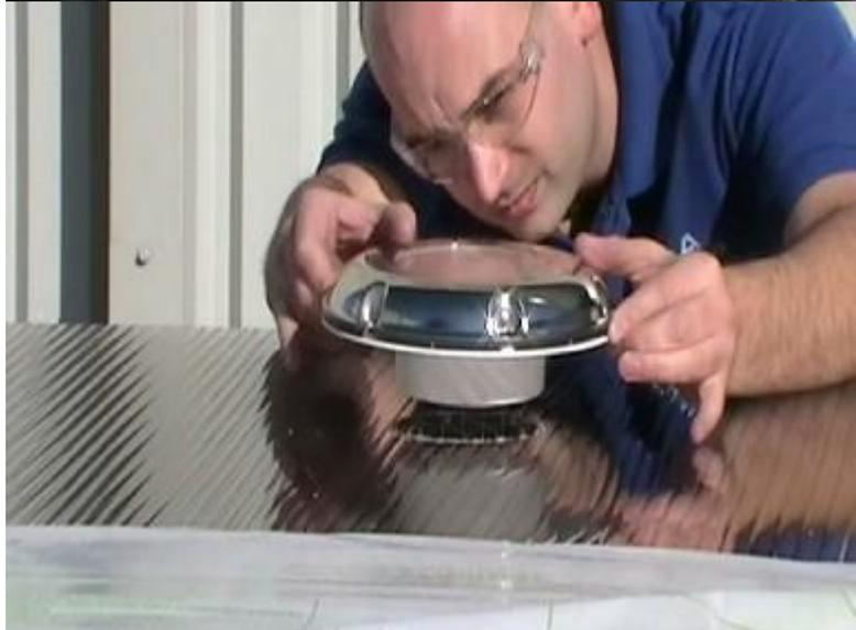
13. Push the solar vent down firmly ensuring a tight seal.
