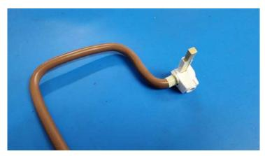
Connect the 16mm tail leads to the schneider feed-in connectors
