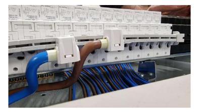
Fully Tighten all connections ensuring everything is tightened to Torque (busbar 2NM, isolator 3.5NM)
