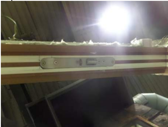
Top latch forend in frame head – doorset B
