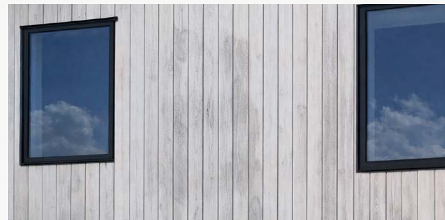
A New Zealand housing project with a distinct batten (sub-frame) silhouette, showing on the cladding surface
