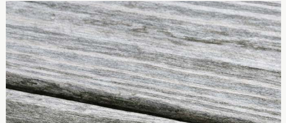
Natural occurring surface fibres on decking
