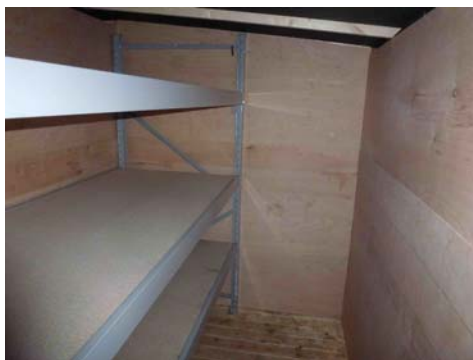
Inside the new storage unit, before our equipment took up residence.
