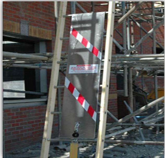
**Figure 1.** A ladder guard that is not wide enough for the ladder it is fitted to. Small feet can still climb the exposed rungs and the guard could slide even further to one side. Narrow ladder guards are only suitable for narrow ladders. No more than 50mm of exposed rung should be visible when the guard is tight to one side of the ladder.
