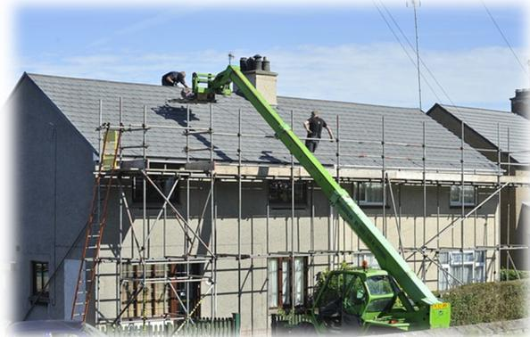
Clients and contractors must ensure that unauthorised access onto scaffolding is prevented, not just outside working hours, but also at times when workers are present but out of sight.
