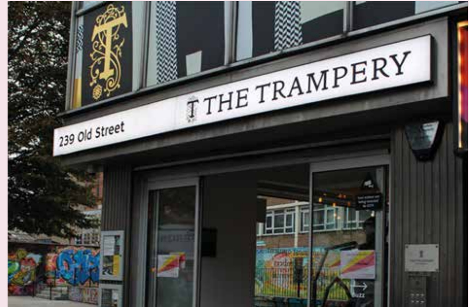
Figure 33. The Trampery, Old Street
