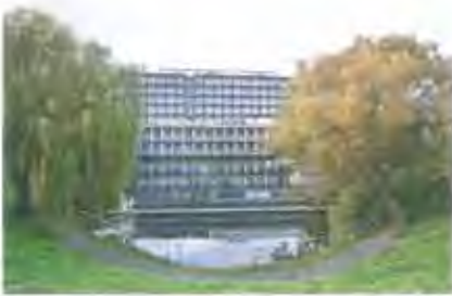
When Usher Architects bought a derelict 1970s office building, CorTen Bristol set out to make the central part of a regeneration area. It has a lot to teach us on how to make the most of an existing building.
