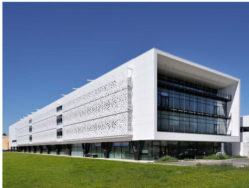
Illustration 1. KRION® EAST® K-LIFE Porcelanosa Solid Surface. Exterior cladding.
