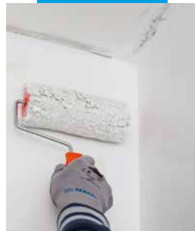
Application of Dursilite Plus with a roller
