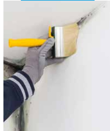
Application of the primer (use preferably Silancolor Primer Plus )
