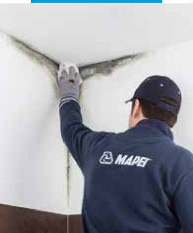
Cleaning the walls with Silancolor Cleaner Plus
