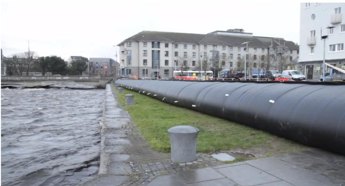
Figure 3-4: Temporary flood defence 7 at Spanish Arch
