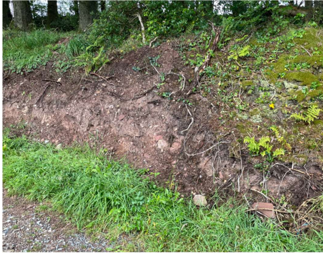
Figure 4-62 Forestry on top of sandy substrate with some gravel-cobble material.
