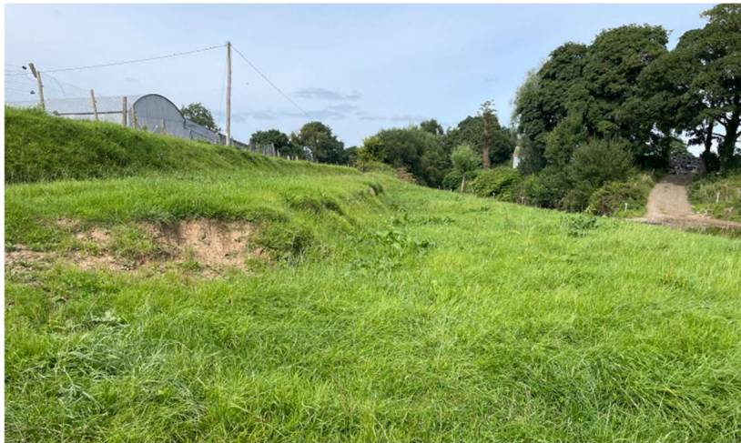
Figure 4-45 Second and third stages of the channel (right bank looking upstream).
