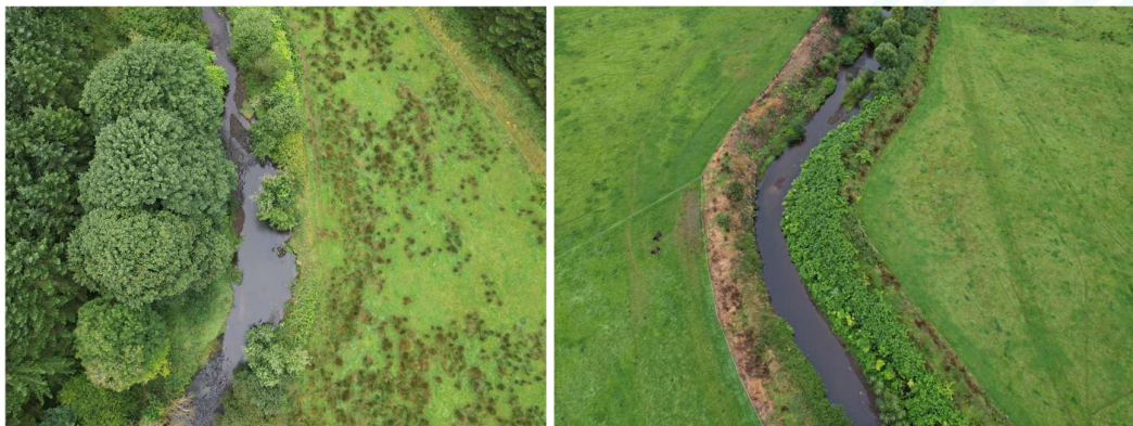
Figure 4-64 Drone imagery upstream from Annagh 4 bridge. Riffle-pool sequence with anabranching flow on bar and fencing to protect riparian strip from horses (not known if this is intentional).
