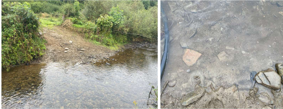
Figure 4-67 Bankside poaching to the River Annagh and Condition of Bed at Location.
