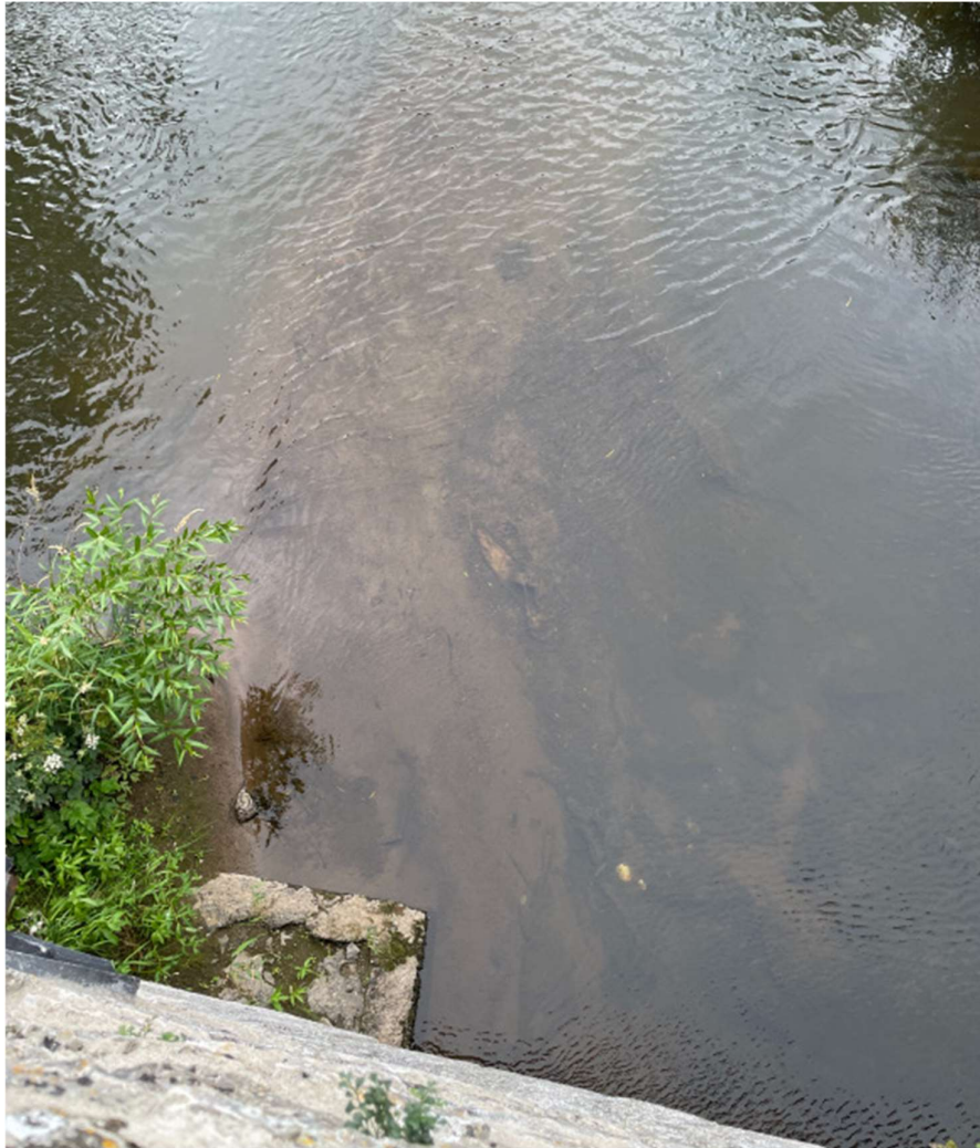
Figure 4-23 Fine sediment bar feature immediately downstream of the bridge. Additionally fine sediment veneer on the channel bed.
