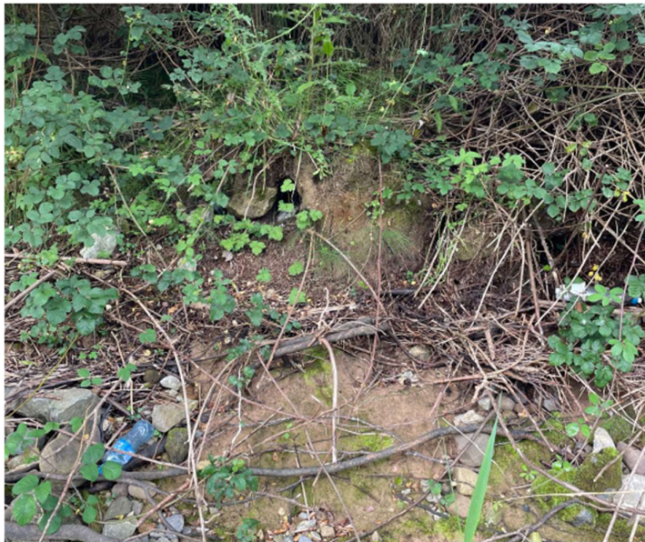
Figure 4-10 Evidence of fine sediment input, exposed roots and silt/sand parcels are visible. (Left bank).
