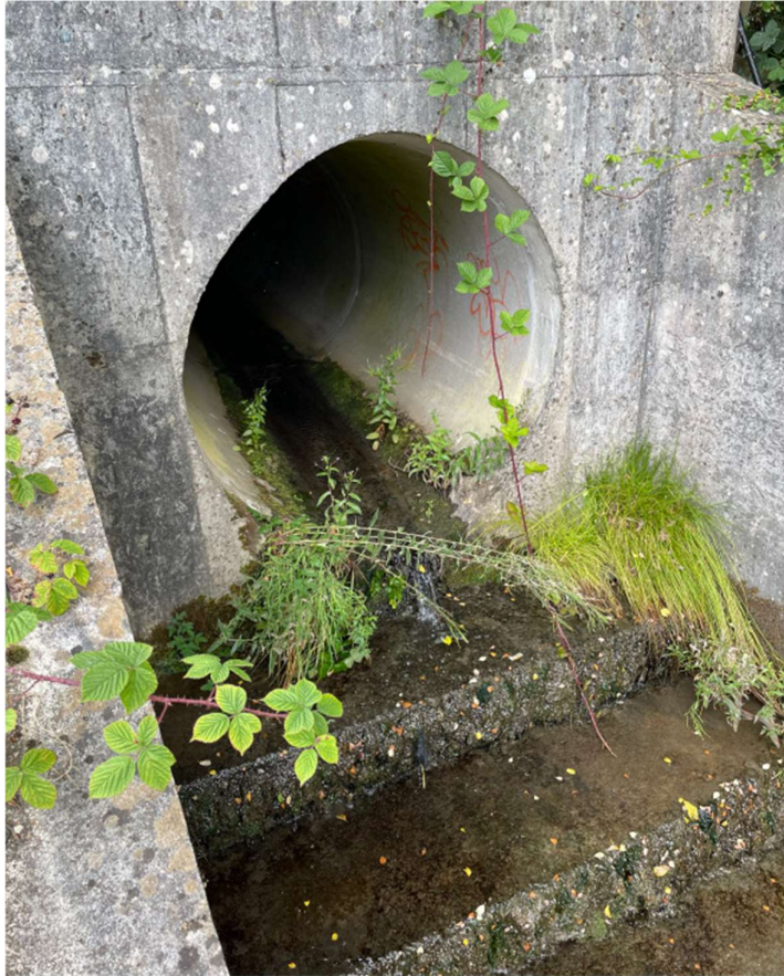
Figure 4-12 Outfall draining into Mulkear 2 downstream from the motorway.
