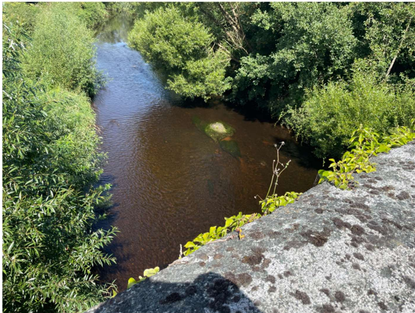
Figure 4-42 Upstream from Annagh Bridge with mid-channel gravel bar and a vegetated bar on the right bank (left of picture).
