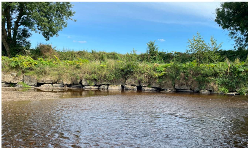
Figure 4-46 Channel reinforcement boulder material (looking across to left bank).
