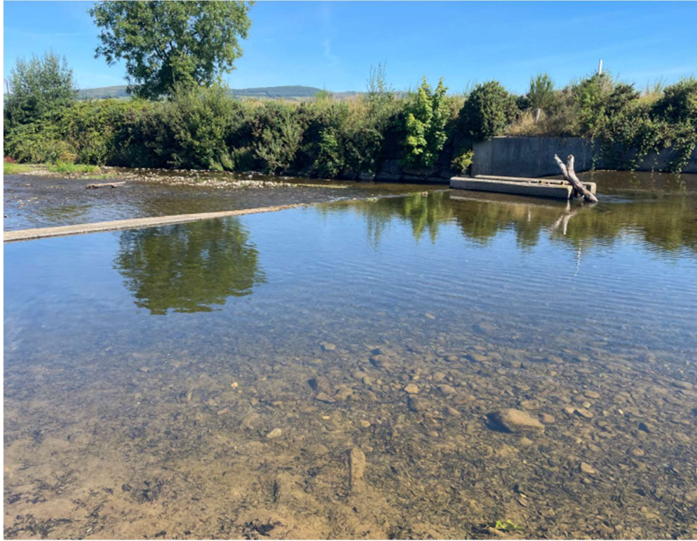
Figure 4-34 Silty material upstream from weir crest and more dynamic flow downstream.
