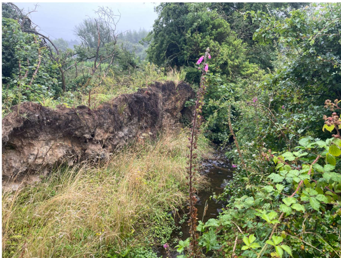
Figure 4-70 Tributary draining into Annagh with fine sediment and incision issues.
