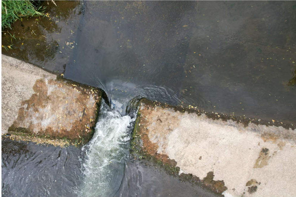
Figure 4-29 Gauging weir crest - coarse sediment slightly below water level upstream.
