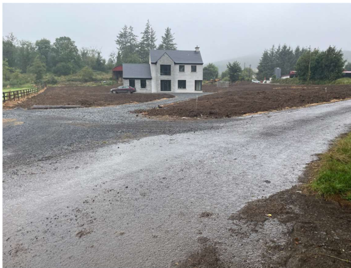
Figure 4-69 Landowner construction works and exposed fine sediment.
