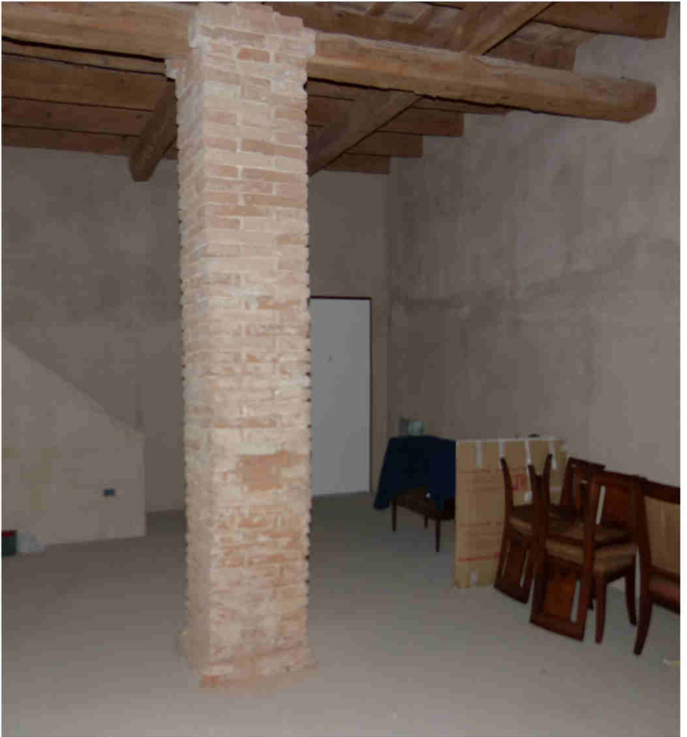
locale al piano seminterrato
