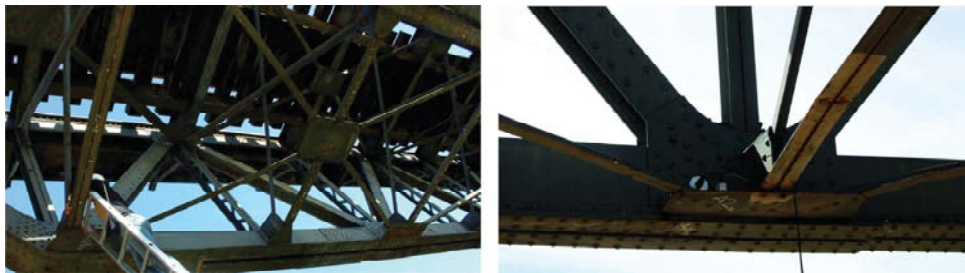
Figure 25: (left) Track in the Bridge over Jabalón River and (right) accelerometer at the truss connection.
