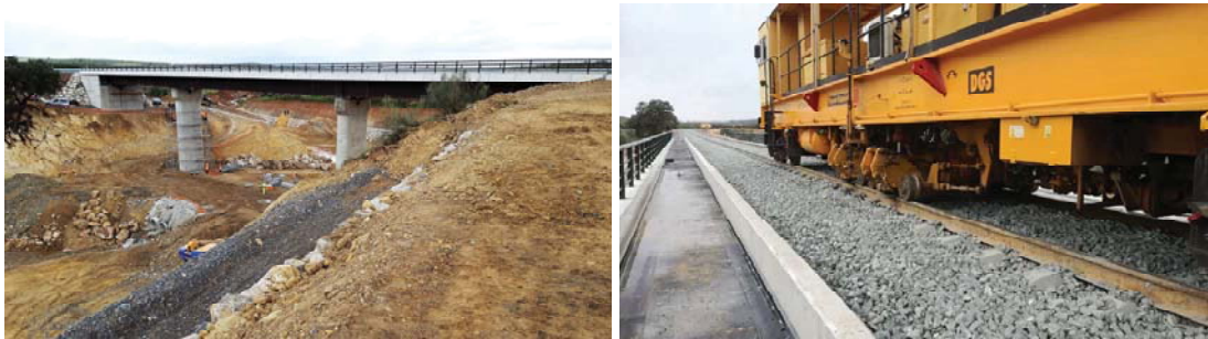
Figure 27: Bridge over Tinajas River ( 37^{\circ}01'41.0''\text{N} 4^{\circ}45'26.6''\text{W} ).
