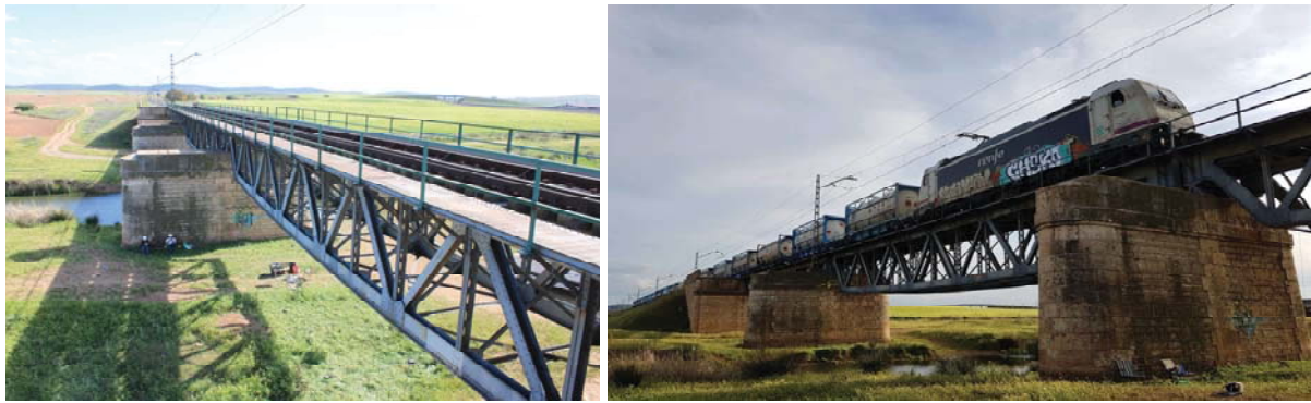
Figure 24: Bridge over Jabalón River ( 38^{\circ}53'51.2''\text{N} 3^{\circ}57'44.7''\text{W} ).
