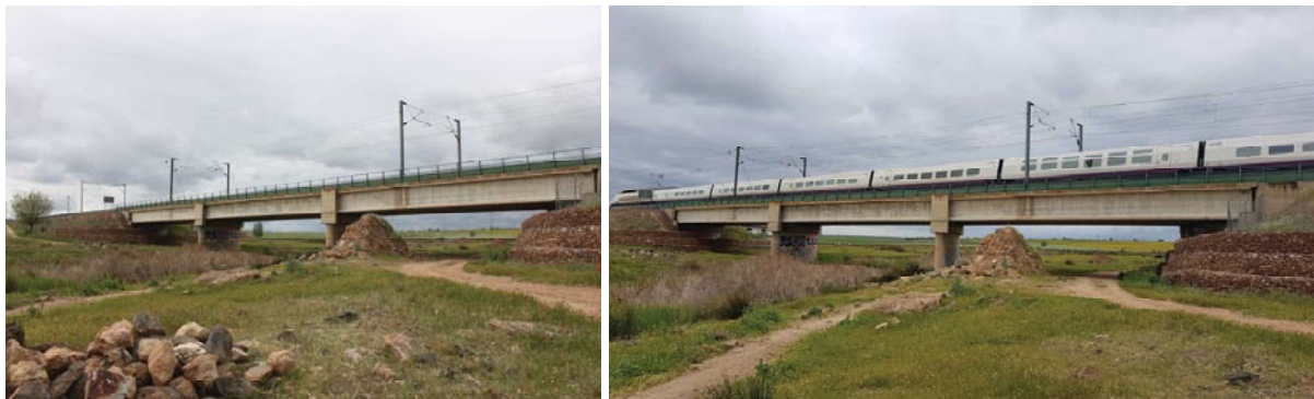
Figure 12: HSL bridge over Jabalón River ( 38^{\circ}53'51.3''\text{N} 3^{\circ}57'53.0''\text{W} ).
