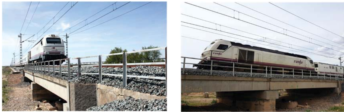
Figure 10: Renfe Altaria Talgo VI trains crossing Old Guadiana Bridge.
