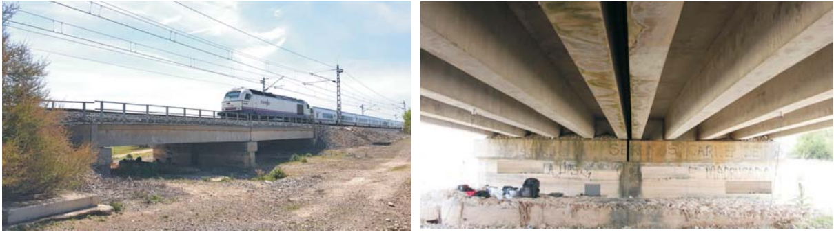
Figure 1: Old Guadiana river bridge.
