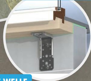
UNI DÜBELANKER MIT WELLE
