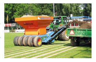
Follow the installation of the secondary drains, a sand top dressing in the region of 100 tonnes would need to be applied to the whole pitch, this being repeated in subsequent years as part of the end of season renovation works.
