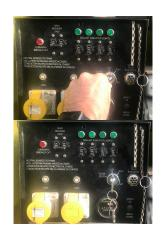
Step 3 Turn the ignition key from the RUN position to the Off position.
