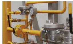
GAS REPAIRS & TESTING
