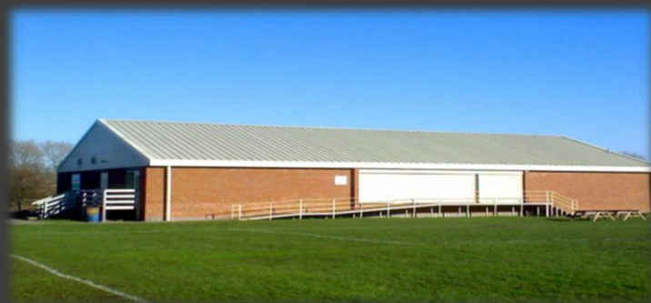
Newly built facilities that include changing rooms, meeting rooms, referees' room, storerooms, physio room, toilets, and bar/kitchen
