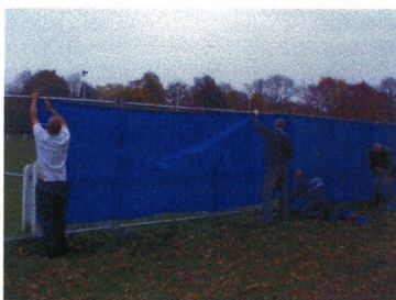
Hire equipment arrives and work begins
