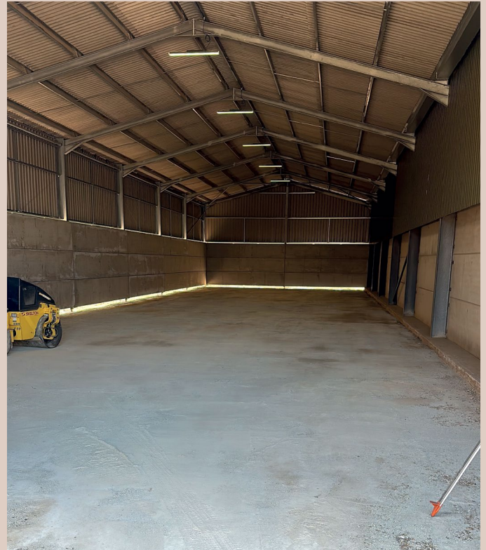
Prepping shed base before laying the floor
