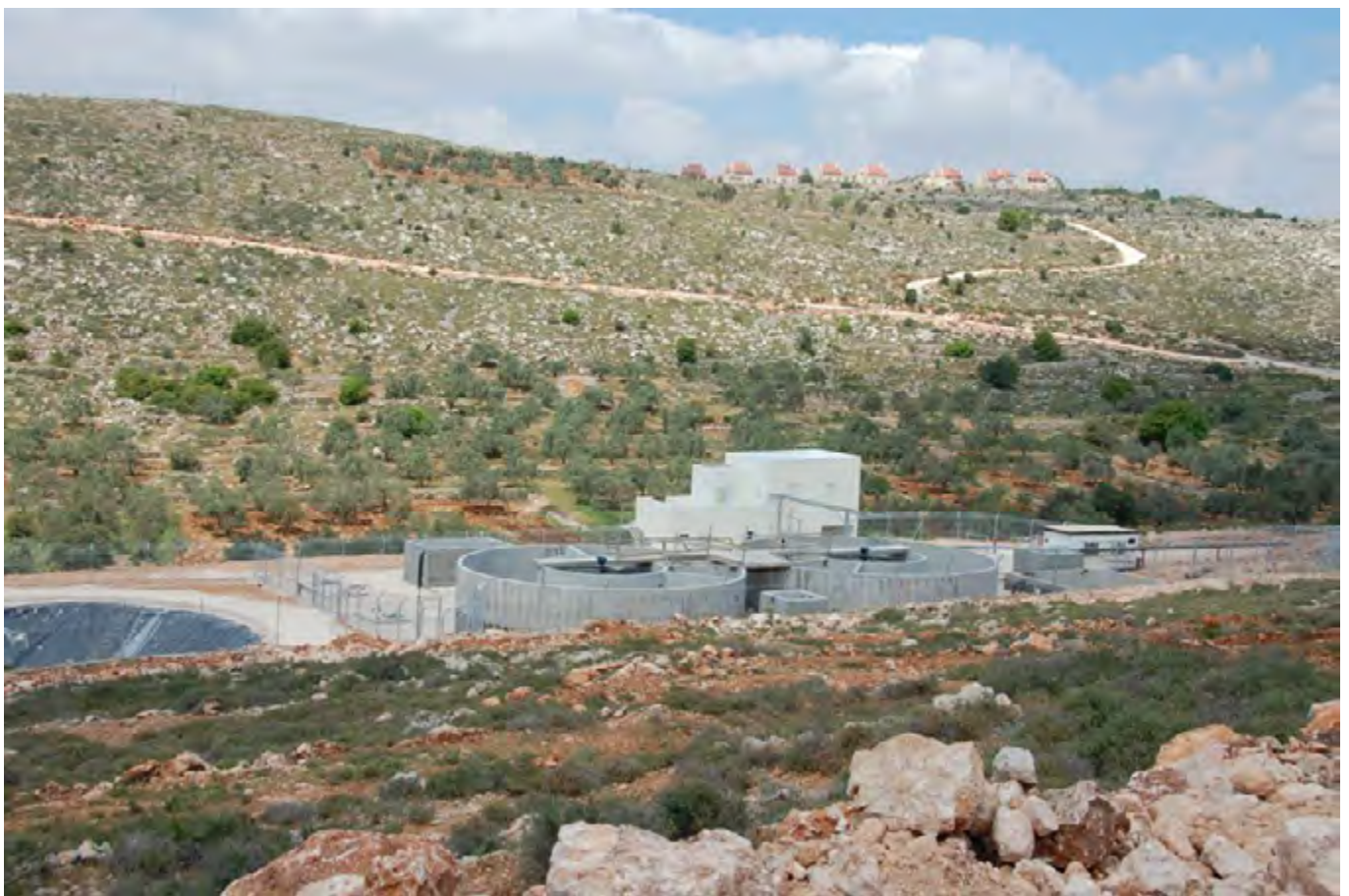
The Ofra sewage treatment facility, built on land belonging to 'Ein Yabrud, March 2013. Israel seeks a formula that would resolve its planning status Photo by Yesh Din
