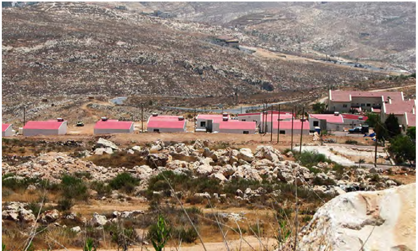
Houses in the settlement of Kochav Ya'akov built on Kafr 'Aqab's land, August 2009. Hundreds of dunams were declared public land in order to avoid removing settlement construction Photo by Yesh Din
