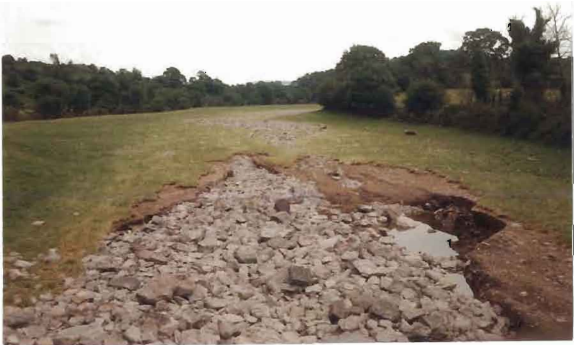
FLOOD RELIEF BRIDGE, UPSTREAM OF MACROOM PHOTOGRAPH NO. 2
