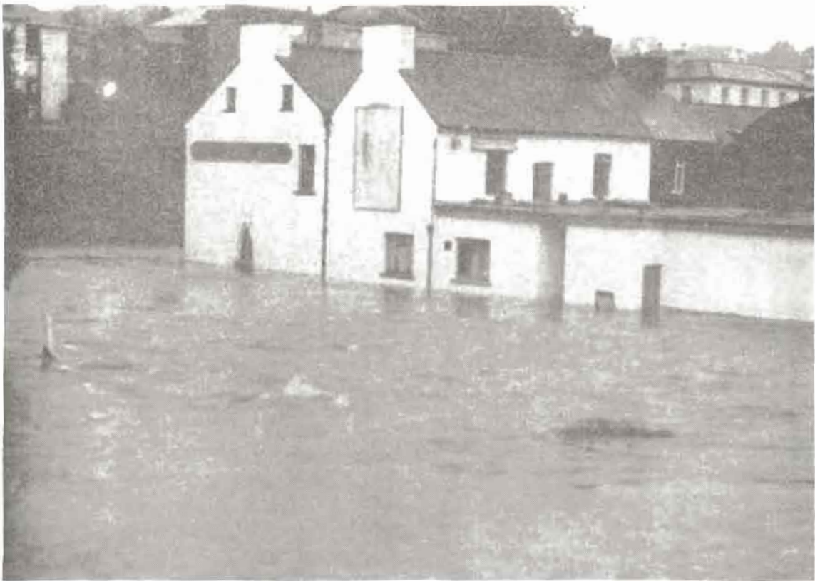
PUBLIC HOUSE DOWNSTREAM OF BRIDGE IN MACROOM TOWN
