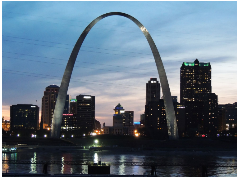
6.34 Der Gateway Arch in St. Louis, Missouri
