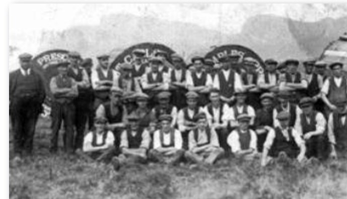
Cable laying gang
