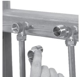
**3** Ensuring adequate provision to allow the water to discharge safely to waste, turn on the supplies to flush the system through. Attach pressure test equipment and pressure test the system in accordance with Water Supply Regulations.
