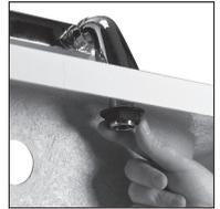
**4** Using suitable connections connect the tap tails to the hot and cold supplies.
