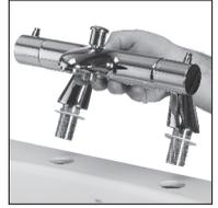
**3** Place the back nuts onto the tap tails and secure the assembly to the underside of the bath.
