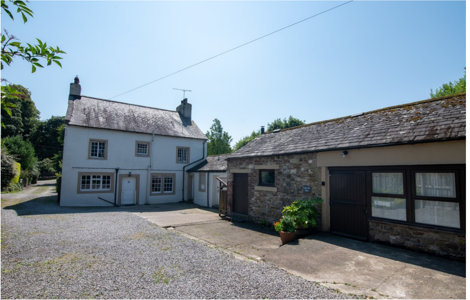
Rear Elevation and Barn
