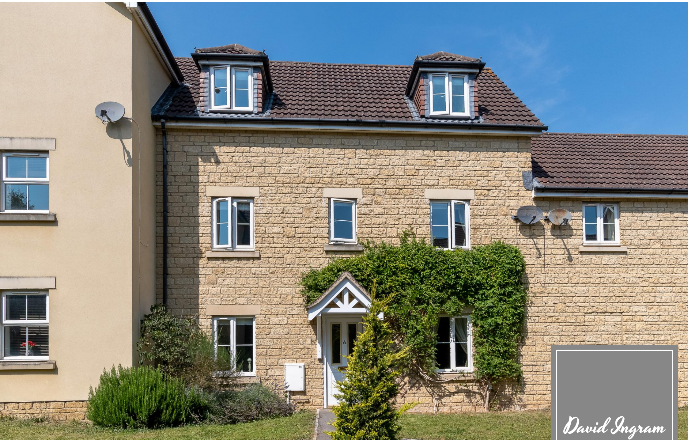
15 Holly Crescent, Corsham, Wiltshire, SN13 9GD
