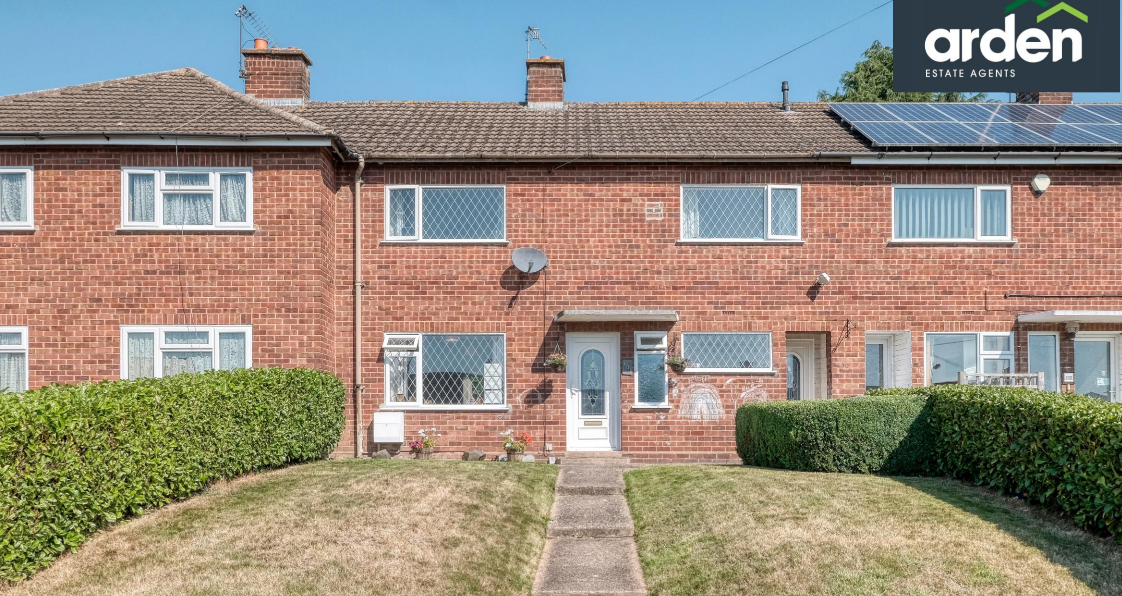
Lyttleton Avenue, Charford, Bromsgrove, B60 3LQ | Offers Over £210,000 Three Bedroom Mid Terraced House
