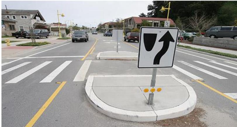
Fig. 11. Median refuges also provide narrowing protection for turning movements and slow traffic.
