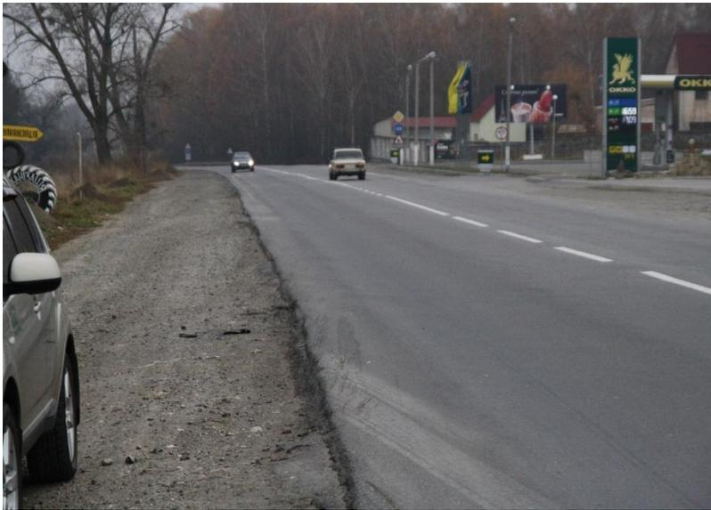
Fig. 9. Shoulder sealing is not current practice – vehicles leaving carriageway, over-correcting crossing to the opposing carriageway and then involved in head-on crashes may be a problem.
