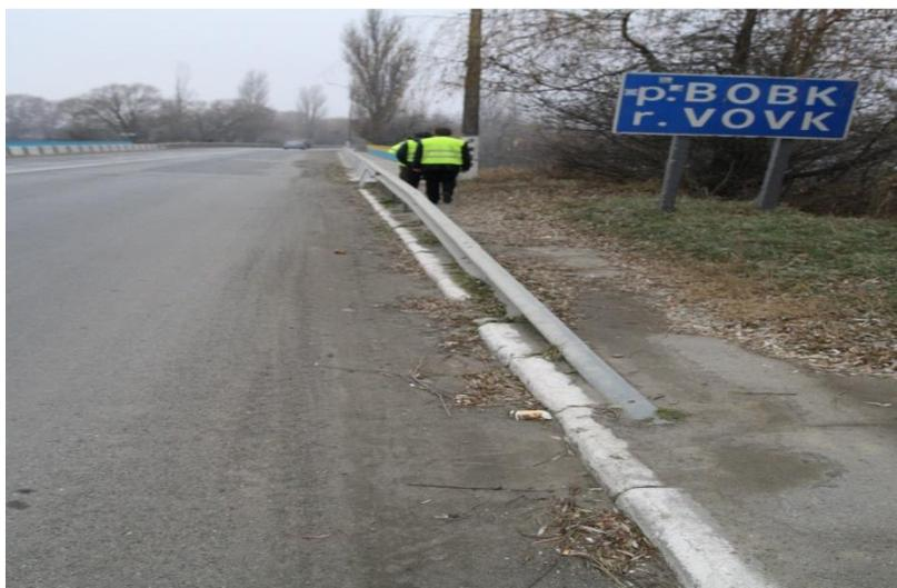
Fig. 7. Continued use of ramped-ends would provide a launch risk for vehicles.
