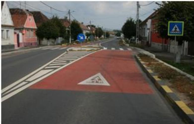
Fig. 12. Changes in horizontal alignment slow traffic and can provide precedence for pedestrians.
