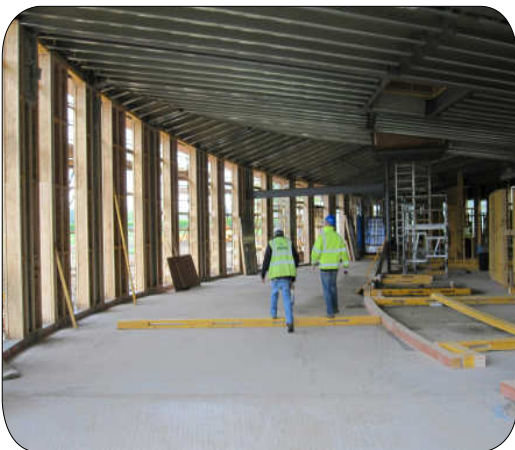
I-Studs forming the curved wall structure
