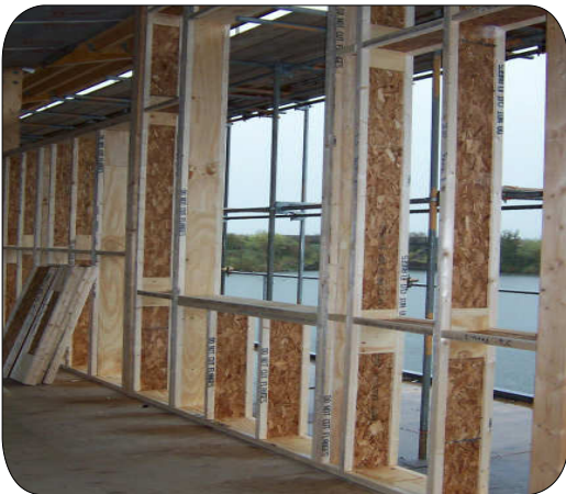
Two storey 300mm I-Studs
