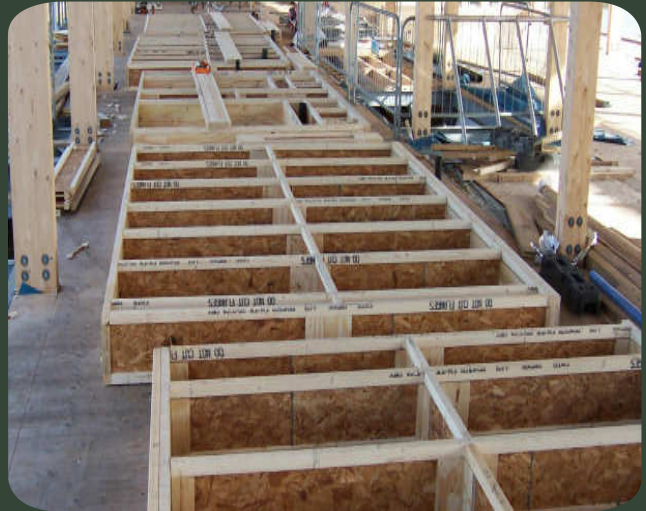
I-Stud wall panels ready for erection
