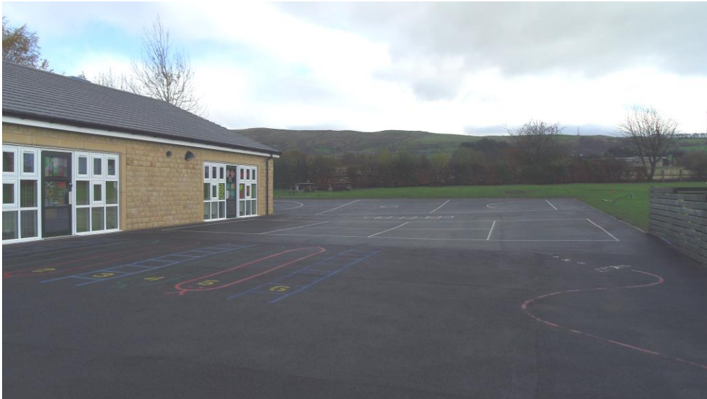
School Playing Fields to rear of School building
