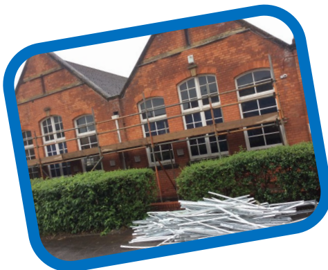
Window replacement - work in progress
